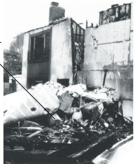
**Figure 10** - The unbraced water heater in this building fell during an earthquake; the resulting fire destroyed the building.
