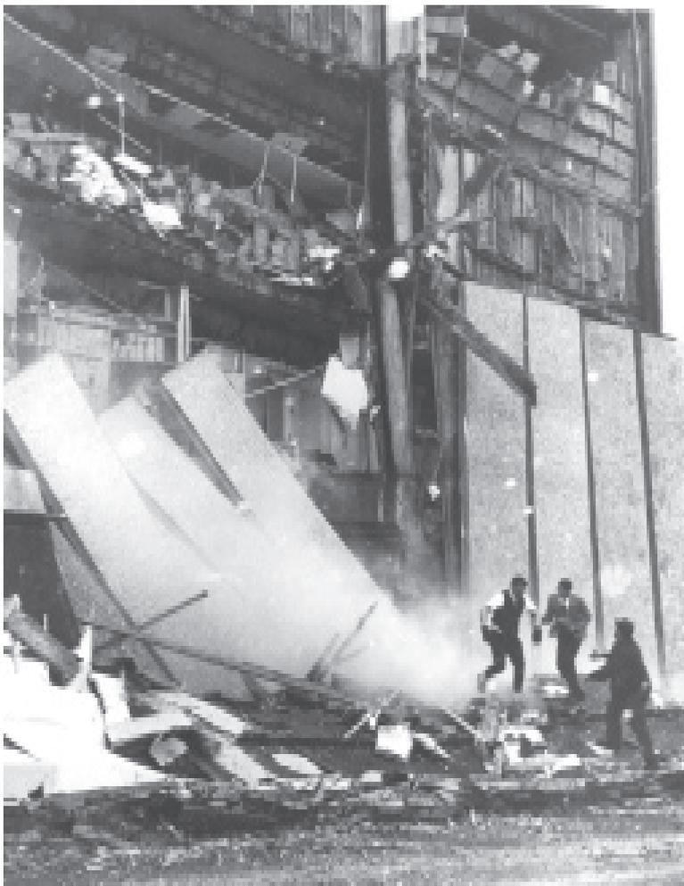
**Figure 37** - Cladding on this store in Anchorage failed in the 1964 Alaska earthquake.
